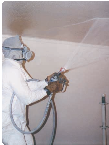
Application by spray accelerates production rates, especially for large projects.
