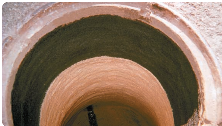
Manhole ChimneySeal prevents inflow through various joints.
